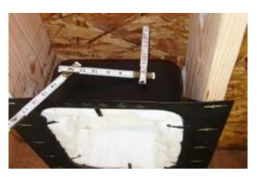
Back Box Installed showing overhead clearance
